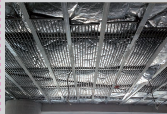
Plasterboard ceiling with metal base
